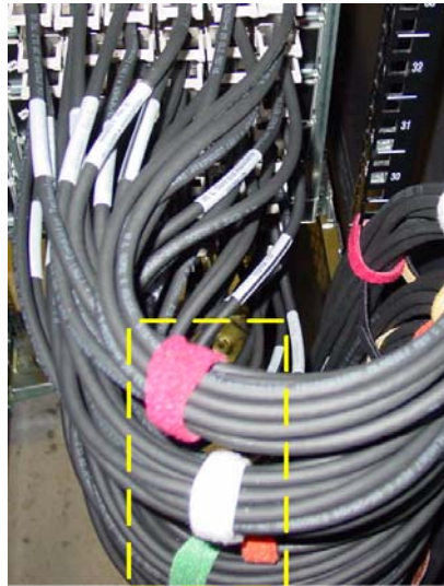
Figure 2-7 Velcro to Bend Radius Midpoint
