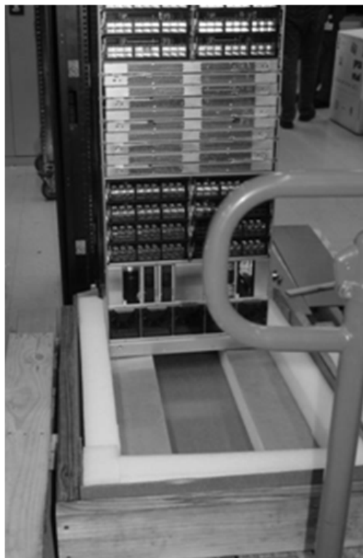
Figure 1-36. Sliding the Switch off the Pallet
